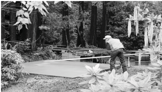
CONSTRUCTION HAS BEGUN ON THE BREAD OVEN
