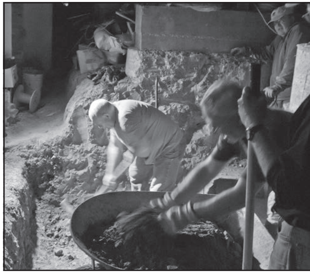
Gualala Arts volunteers dug the new elevator shaft by hand.
